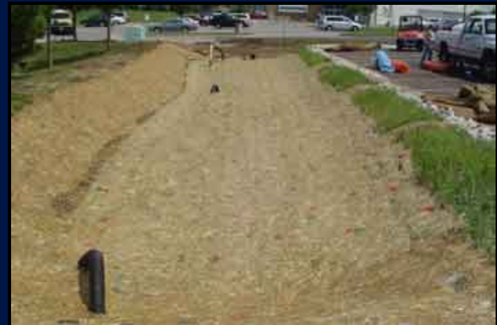
Planting of an Overland Park, KS bioretention cell Photo courtesy of Johnson County Stormwater
